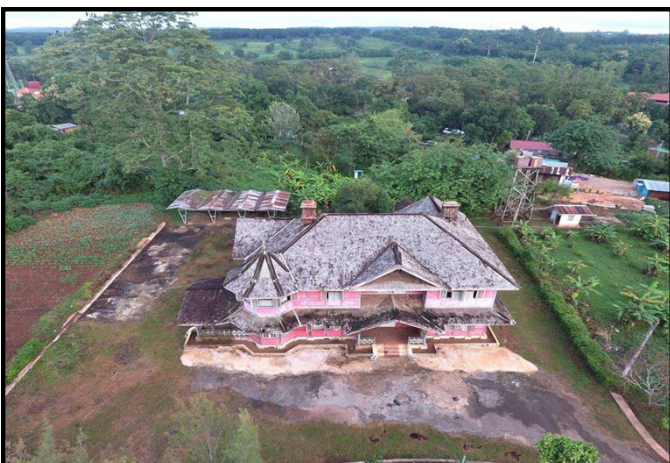
Ancient Yuzanamyaing Tatmadaw guesthouse (before renovation)
