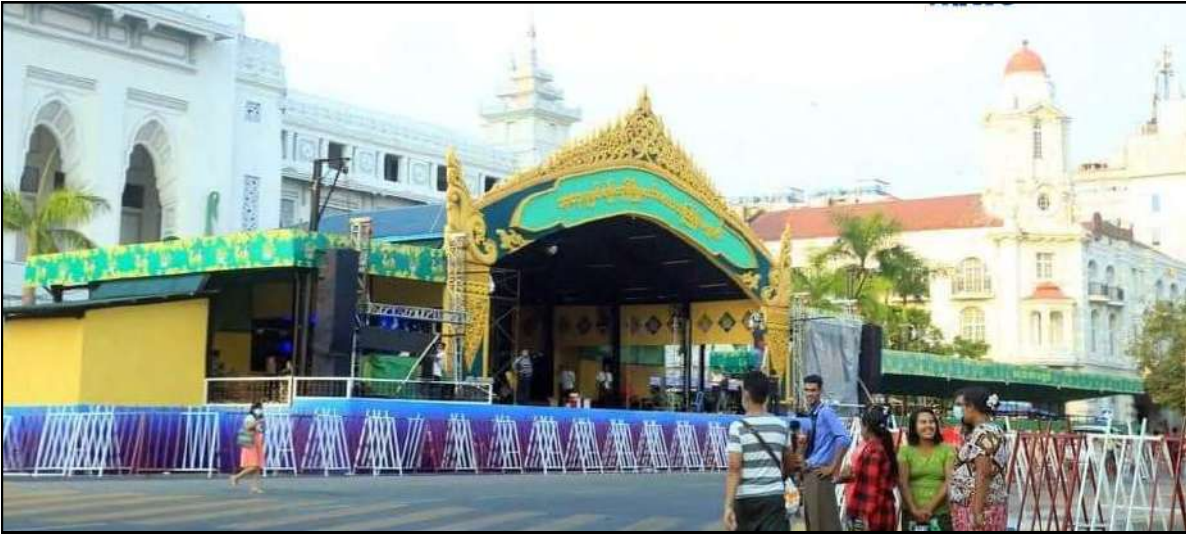
Construction of Yangon Mayor Central Pandal
